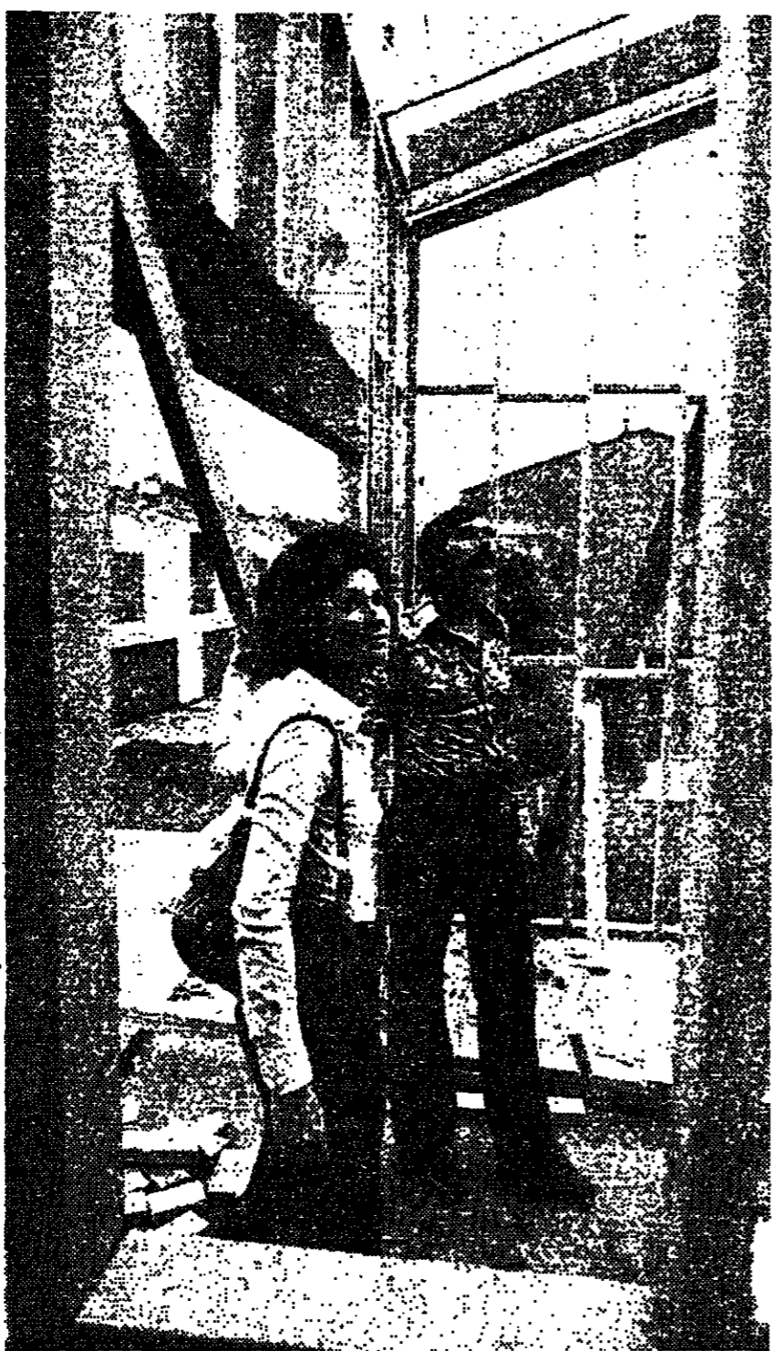
Betty and Eric Young check on condominium they are building. They hope it will be ready next month.
